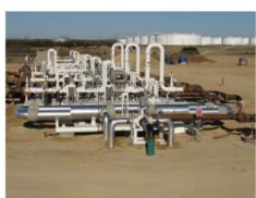
A comparison can be made between the cycle time of either the Coriolis or Ultrasonic and the length of the prover calibrated section. From experience we have found a minimum of ten seconds from switch to switch produces an acceptable repeatability that are in line with the API requirement of five round trips with less than 0.05% deviation between the round trips.
