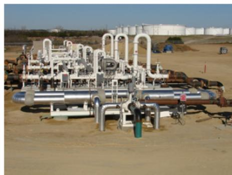
A comparison can be made between the cycle time of either the Coriolis or Ultrasonic and the length of the prover calibrated section. From experience we have found a minimum of ten seconds from switch to switch produces an acceptable repeatability that are in line with the API requirement of five round trips with less than 0.05% deviation between the round trips.
