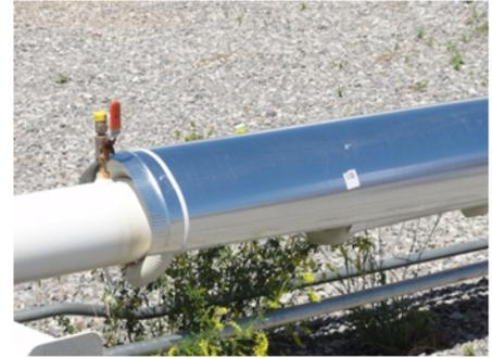
The effect of radiant heat from the sun can be minimized with the use of a sun shade over the metering equipment. Insulation works also but insulation works both ways, it can reduce the effect of radiant heat but it also traps heat as the equipment and process are trying to stabilize.
