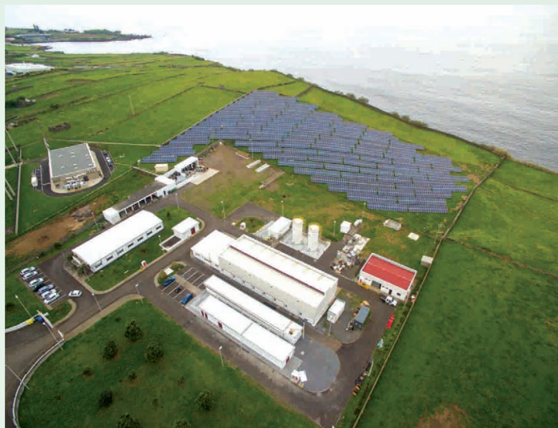
Hybrid energy solution on the island of Graciosa in the Northern Azores region of Portugal
